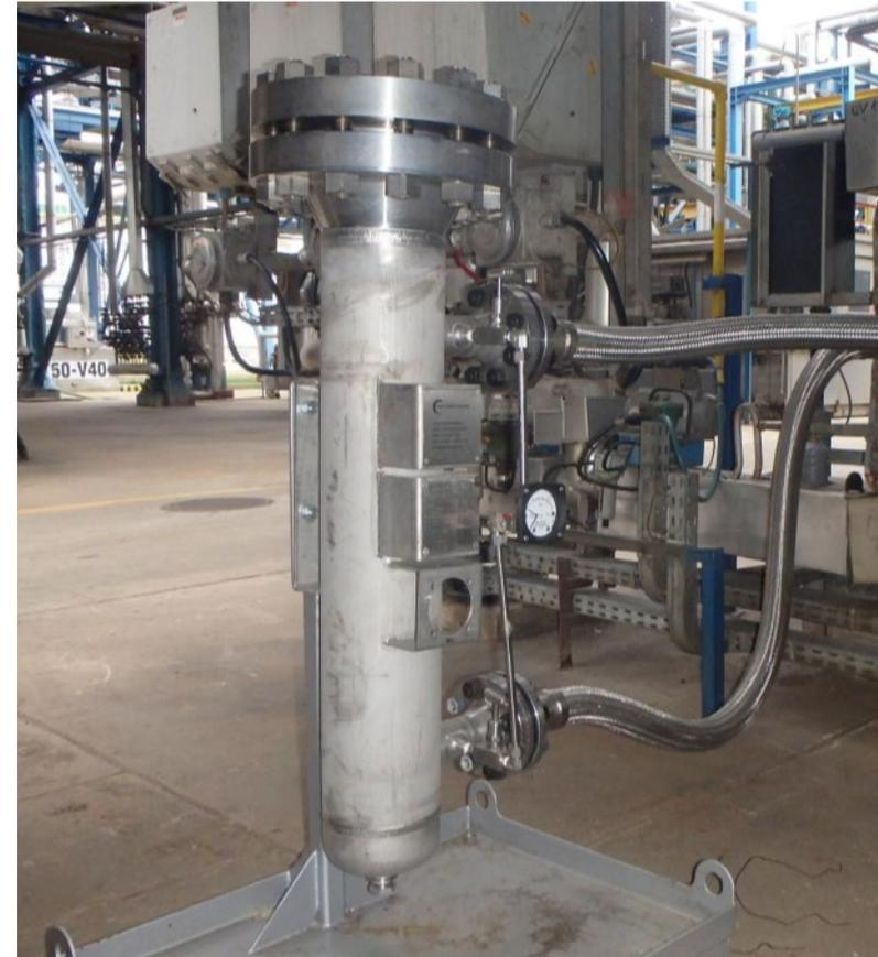
BPS magnetic separator installed in the fuel gas system of the hydrocracker complex.
